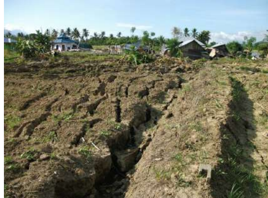
Figure 3.15. Massive ground crack direction north-south from the earthquake caused residents' houses damaged in Jono Oge area, Sigi Biromaru District, Sigi Regency, on September 28 th , 2018.
