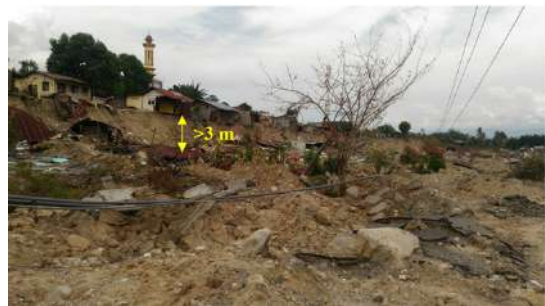
Figure 1.2. Road subsidence exceeding 3 m on the landslide crest caused by liquefaction in the Balaroa area.
