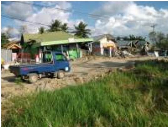
Figure 3.14. The ground oscillation caused buildings damaged by the earthquake in Jono Oge area, Sigi Biromaru District, Sigi Regency on September 28 th , 2018. Earthquake intensity scale reaches IX MMI in Jono Oge area.
