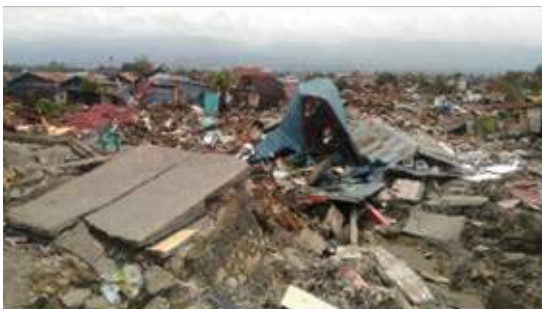
Figure 1.5. Damage caused by flow-type liquefaction phenomena.
