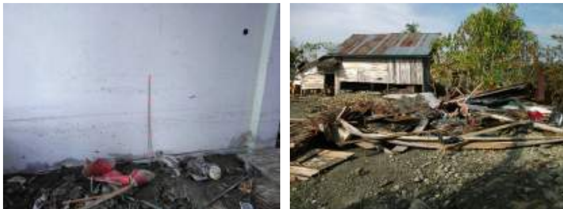
Figure 3.8. Tsunami trace at IAIN campus in Palu City with the flow depth of 1 m (left), and on Sirenja District, Donggala Regency with the flow depth 2 m (right).
